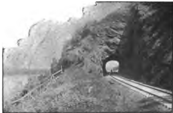
MORRISEY TUNNEL ON THE INTERCOLONIAL RAILWAY, RESTIGOUCHE COUNTY, NEW BRUNSWICK.
